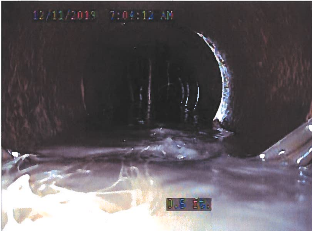
Figure 7: Single wall HDPE to VCP.
