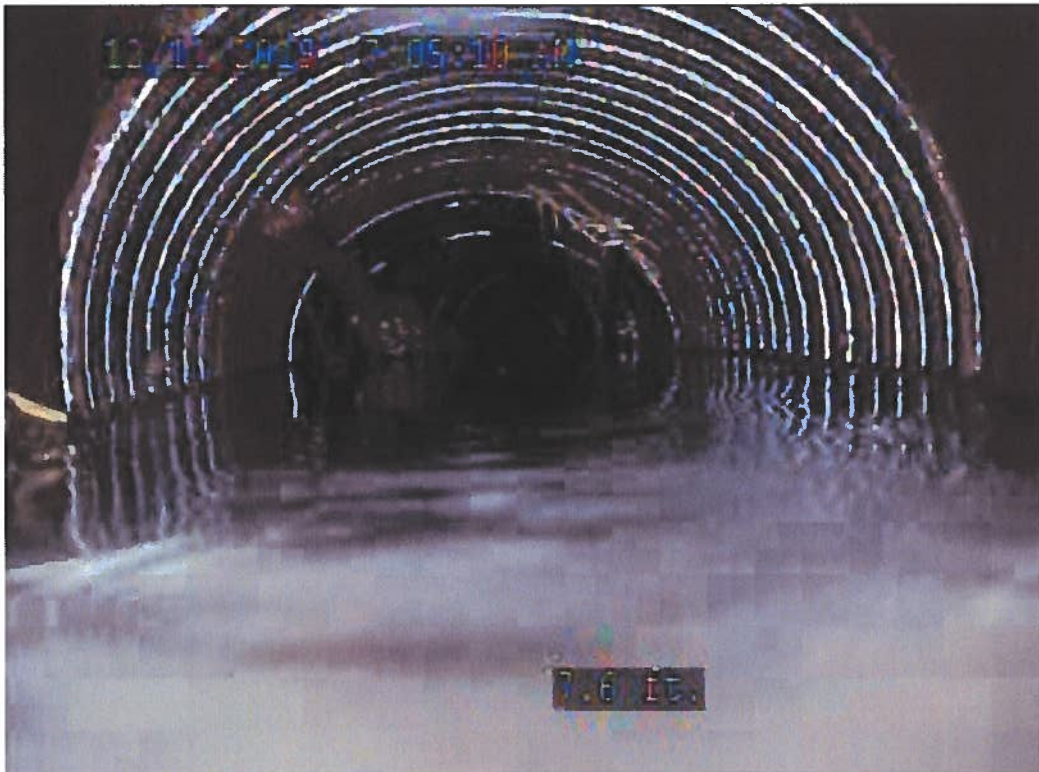
Figure 10: VCP to single wall HDPE.
