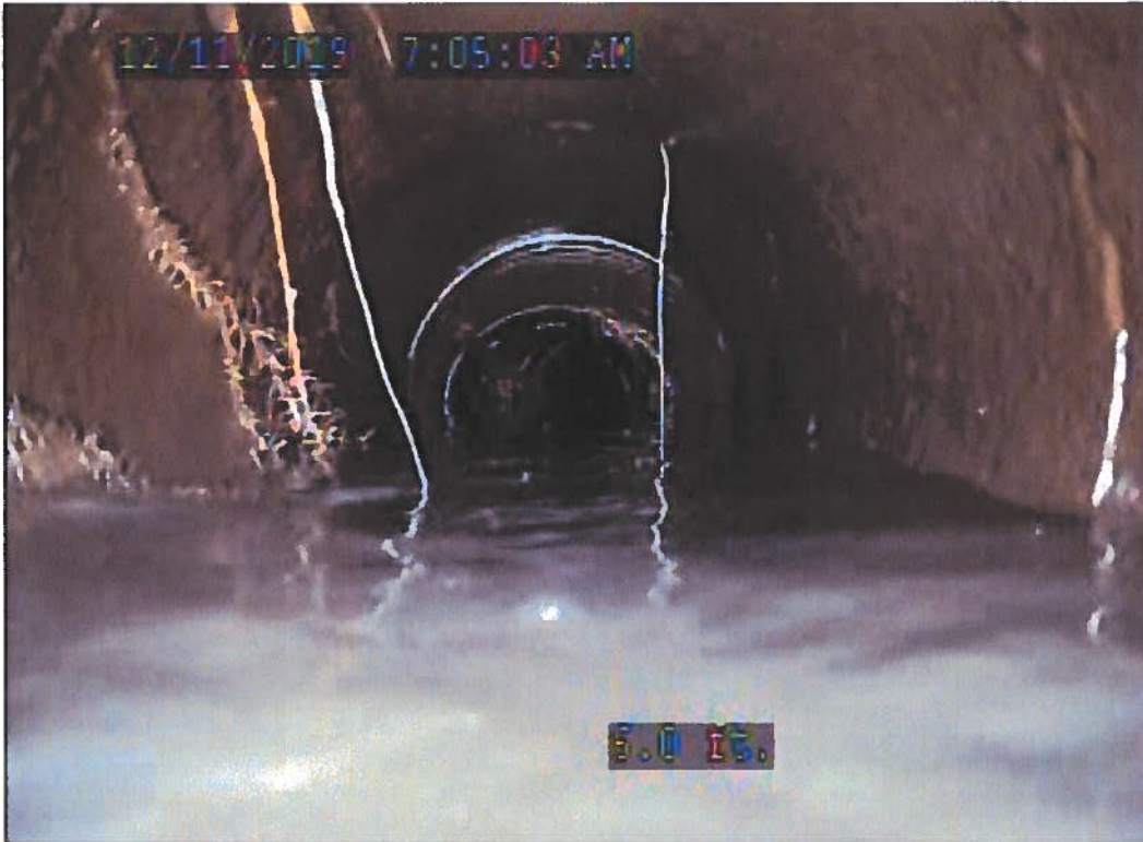
Figure 9: Intermittent roots.
