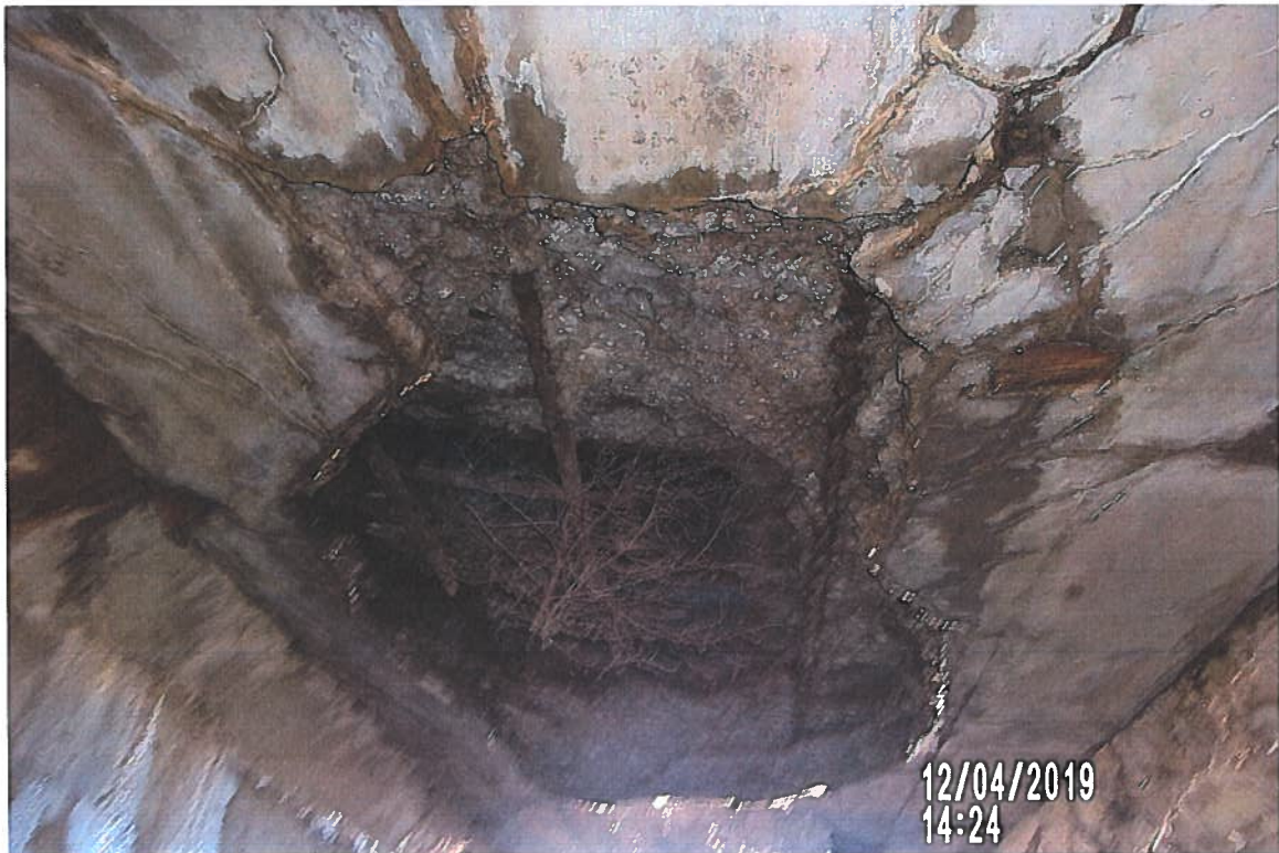
PICTURE # 2461 HOLE IN TOP BOX CULVERT
