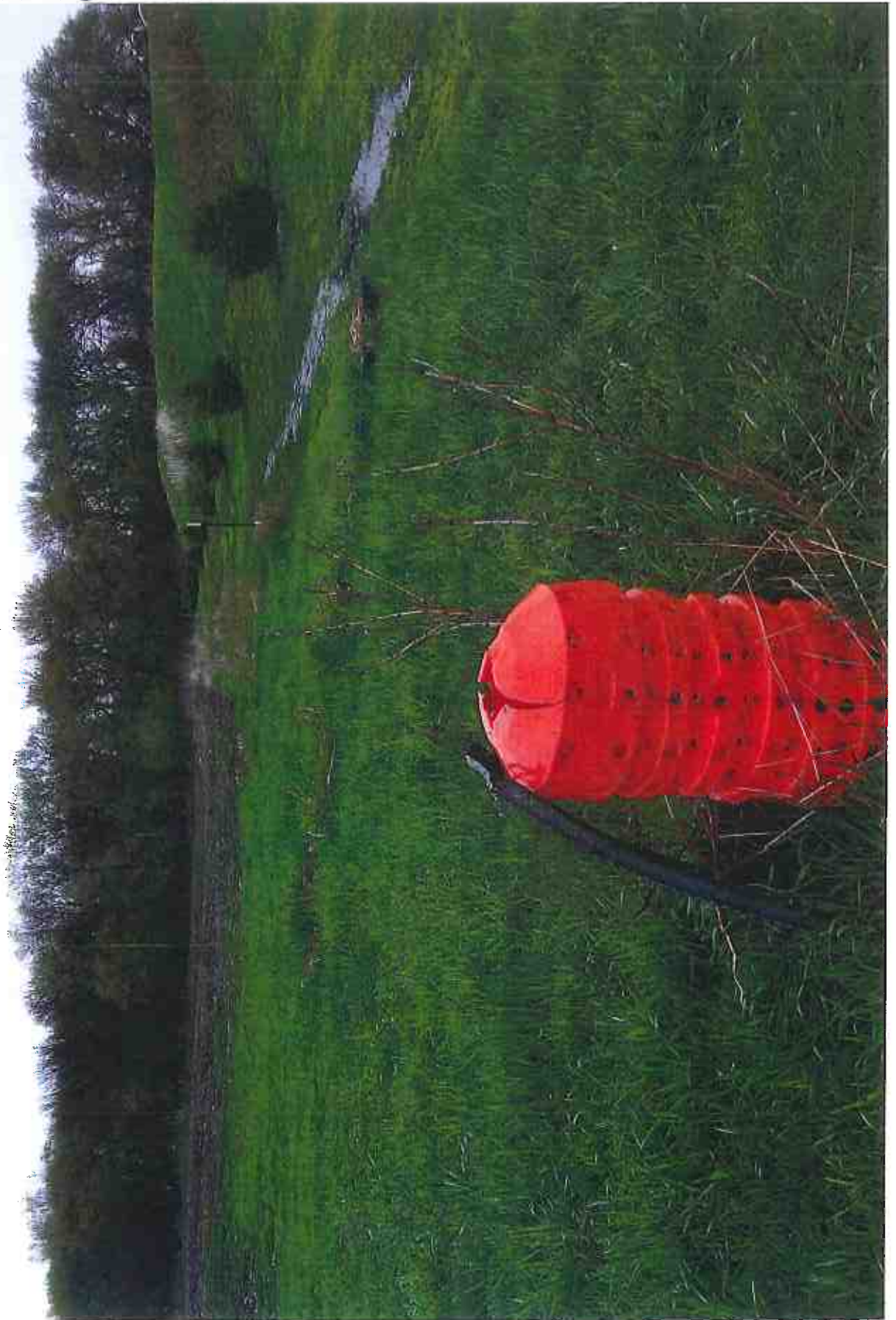
12" HICK INTAKE FULL OF WATER, SWIRLING
