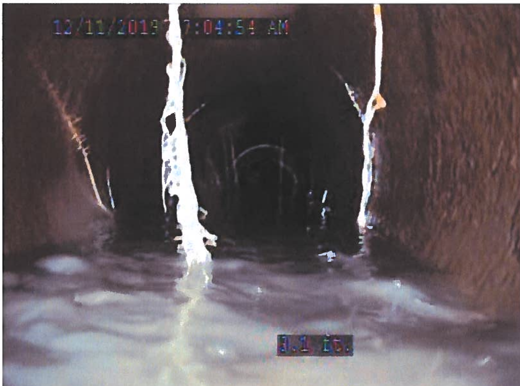
Figure 8: Intermittent, light roots.
